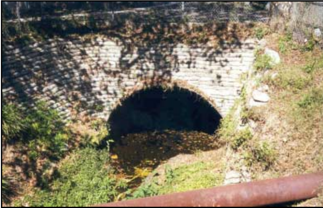
Figure 3.1-2. Private Crossing of Spring Branch Near Betty Lane (to be Removed)
