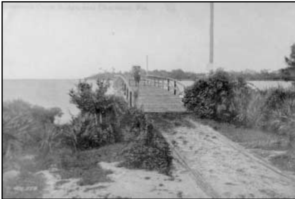
Figure 1.3-2 Stevenson Creek Bridge, near Clearwater, Fla., 1890.
