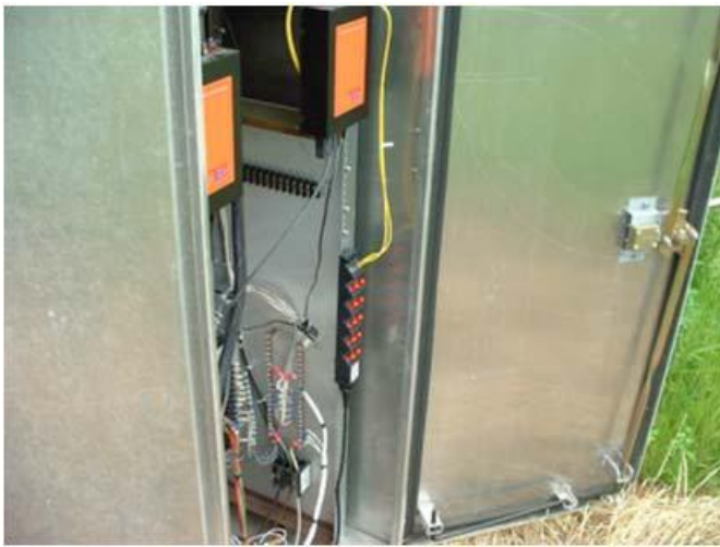
Above photo shows a GatorPatch installed in a typical traffic control cabinet. The blunt (pigtail) end of the cable is spliced to the main underground trunk cable
