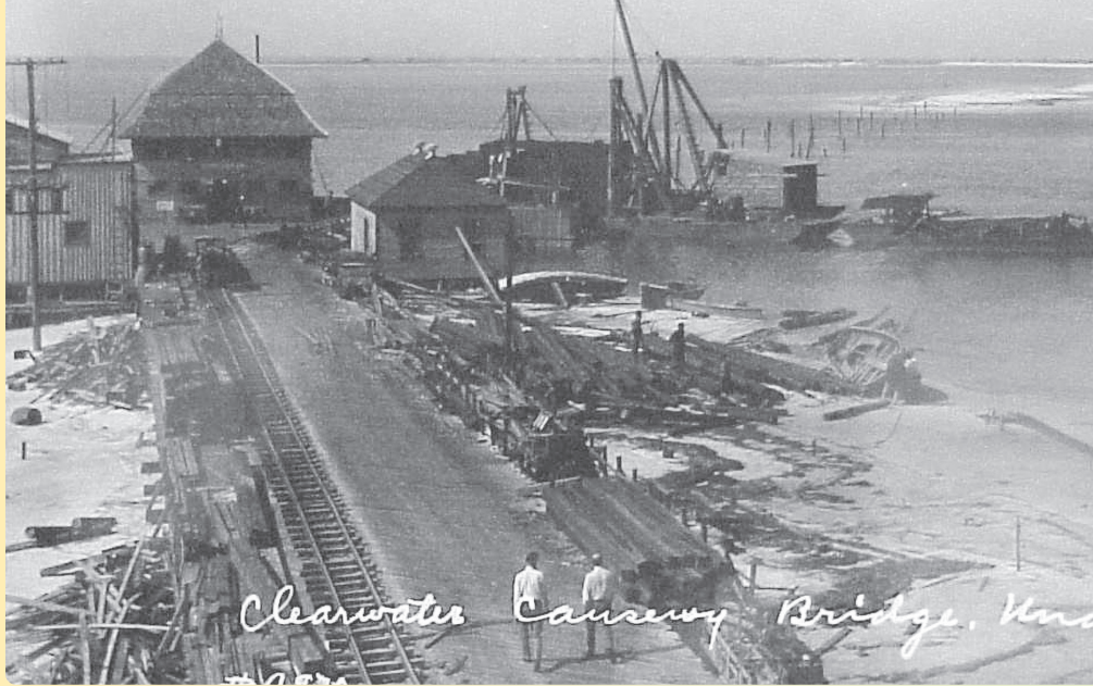
Construction of the Memorial Causeway bridge leading to Clearwater Beach.
