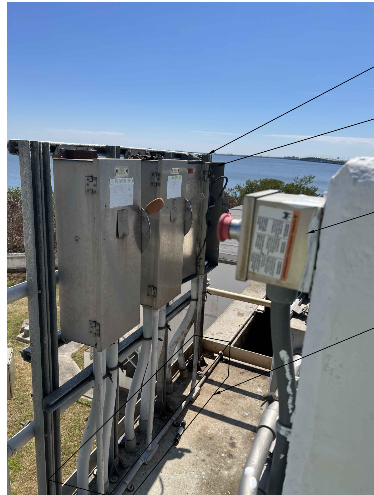
PHOTO: EXISTING SAFETY SWITCHES
