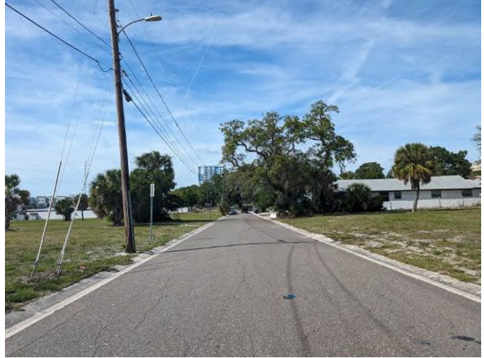
View Looking North Along S Washington Ave (Subject on Left)
