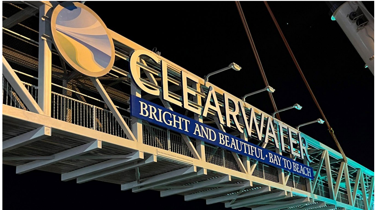
Harn Boulevard pedestrian overpass being installed
