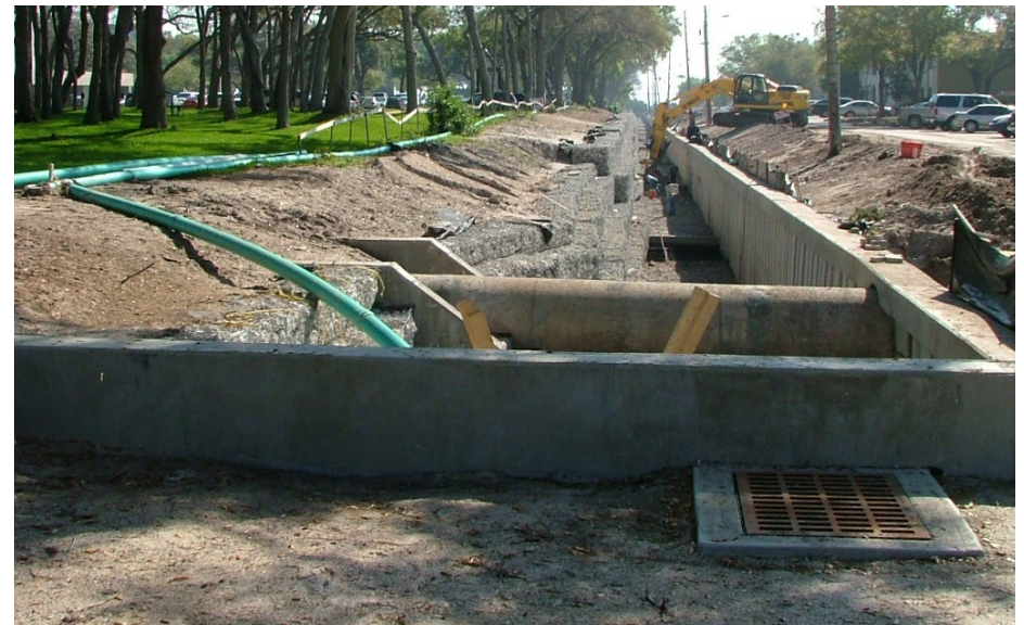
Construction of a stormwater system
