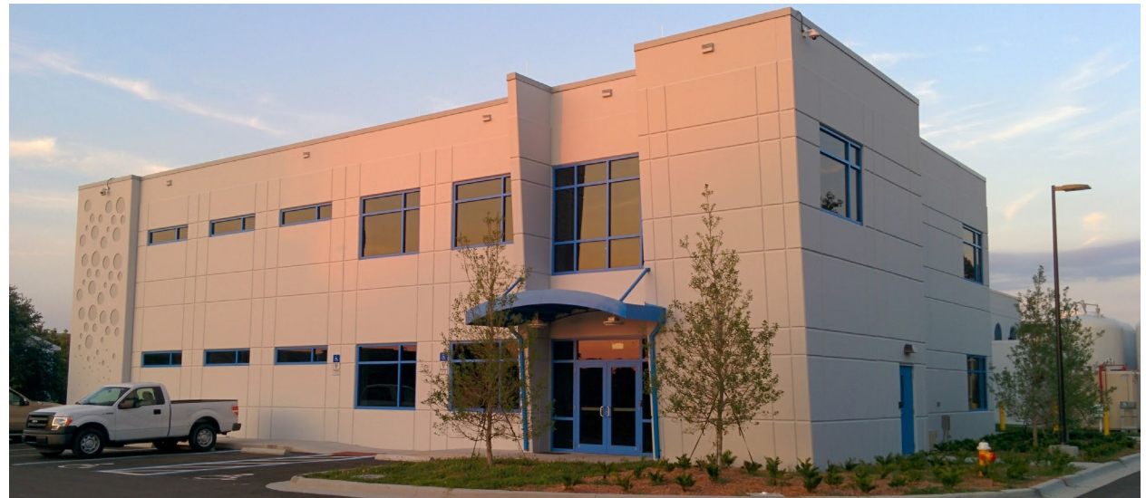
Reverse Osmosis Plant #2
