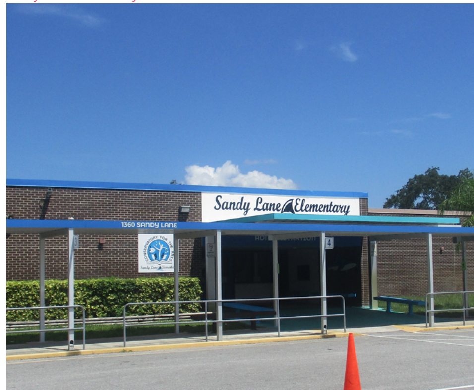
Sandy Lane Elementary School
