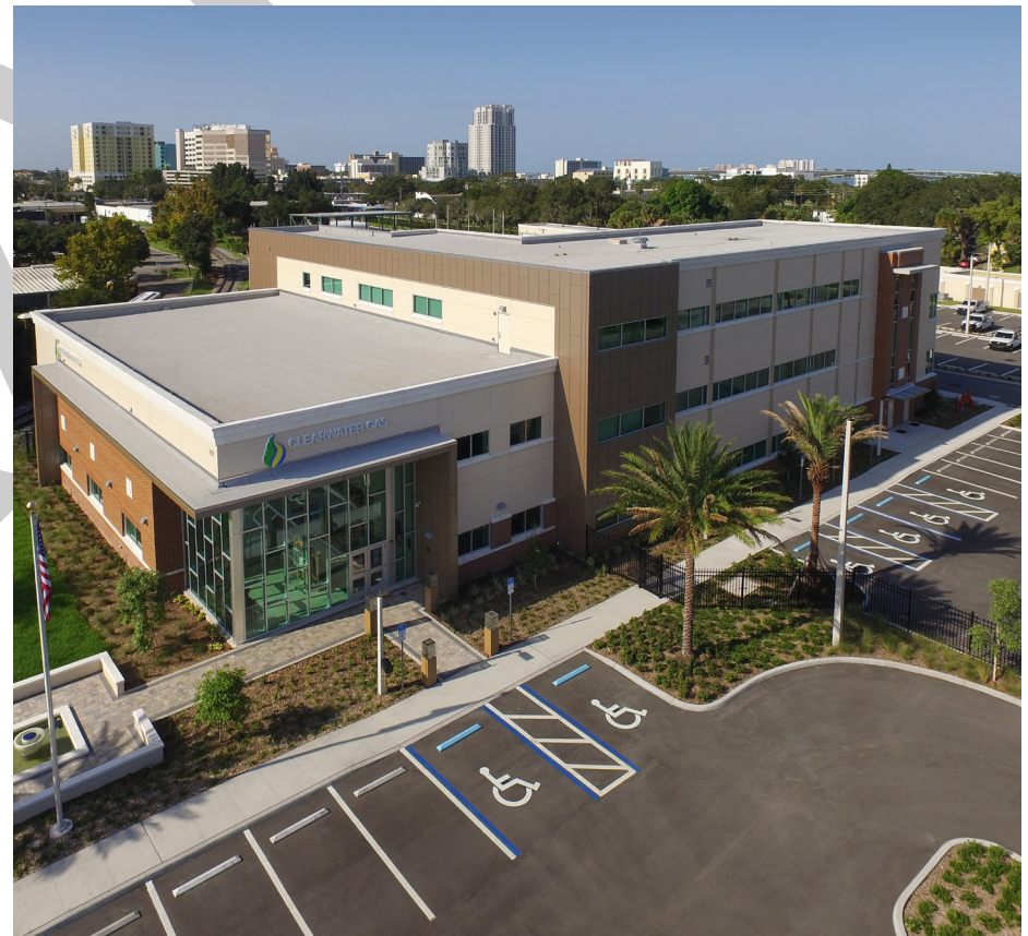
Clearwater Gas Administration Building
